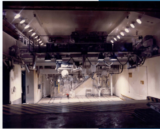
Remotely controlled cranes are used to perform all work inside the canyon.
