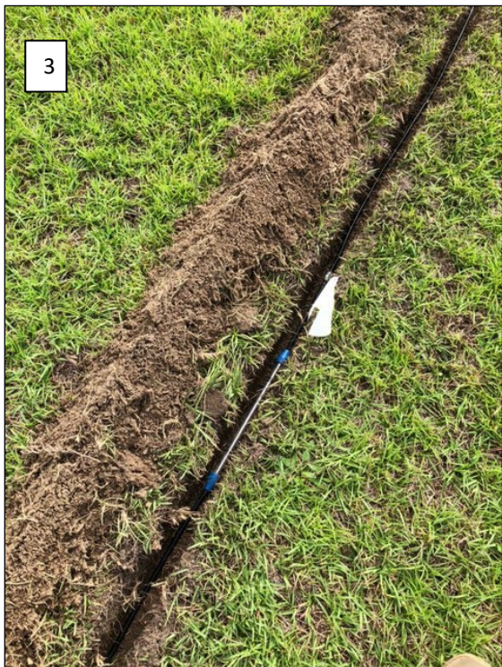
Figure 3-4 Installation of ERT Electrode Cables
