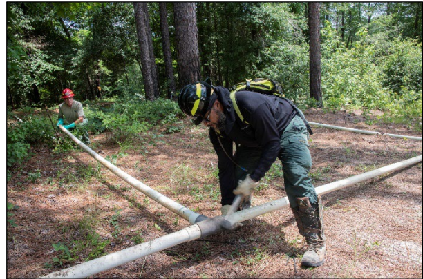
SRS Pines Phytoremediation Project
