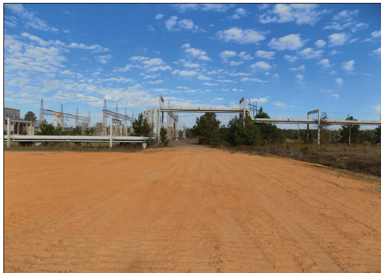
D-Area Coal Handling Shaker House (484-24D) after Decommissioning (Looking North)
