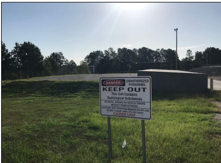
Final View of the SSTs
