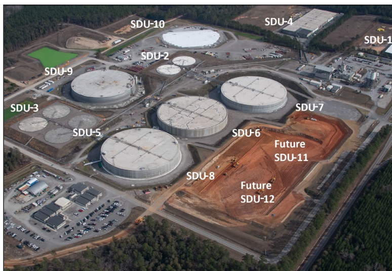
Construction in Progress on SDU-8, SDU-9, SDU-10, and SDU-11
