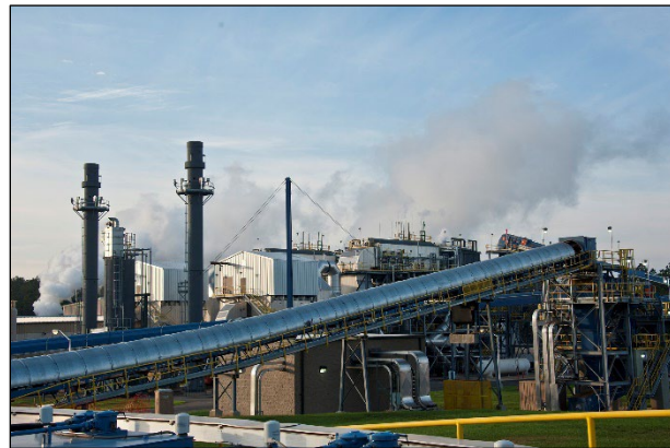
Biomass Cogeneration Facility
