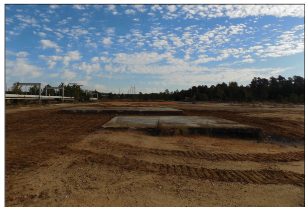
D-Area Coal Handling Crusher House (484-22D) after Decommissioning (Looking East)
