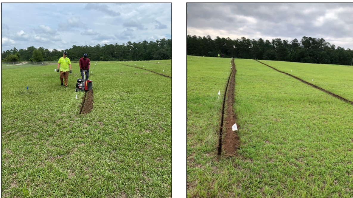
Figure 3-3 Trench Installation to Bury Electrode Cables
